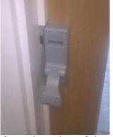
instructions state. If the instructions state fit the push pad 5mm from the edge of the door, then this should be increased by the depth of the rebate (usually 12mm). BUT this needs to be checked before fixing the push pad to the door. Please add a note to the assembly ironmongery fitting box for the position to be checked before fitting.
